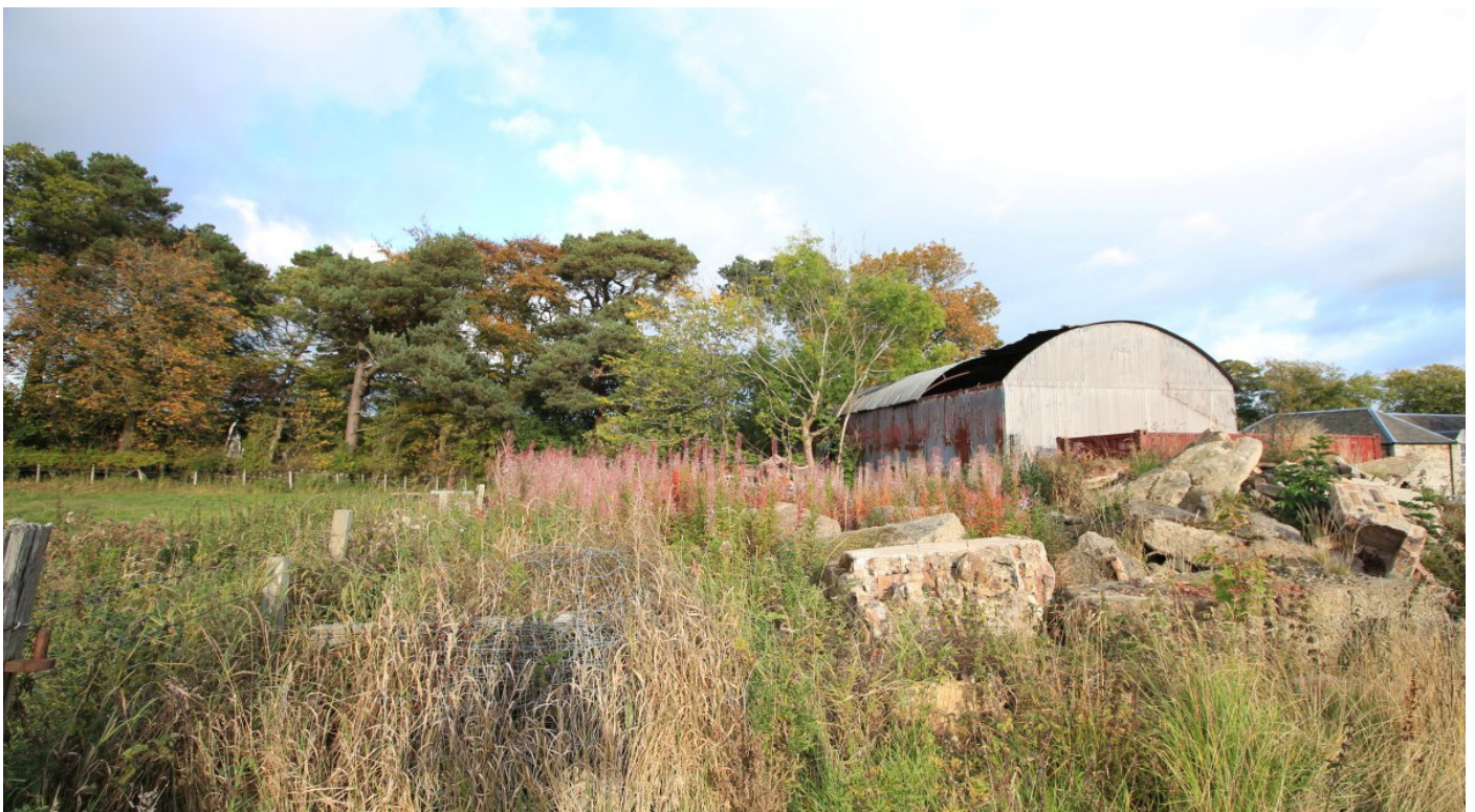
Fig.6 - View of Barn from W
